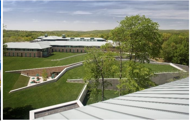
Becton Dickinson Campus Center, Franklin Lakes NJ 11
